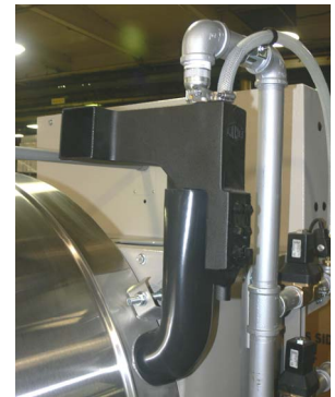
Safe chemical injection
